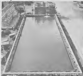
WITHOUT THE refinery background, the reservoir and filter plant north of the Shops appears to be an inviting swimming pool complete with diving platform and shade tree. The reservoir was originally built in 1925 to supply water for several field boilers.
